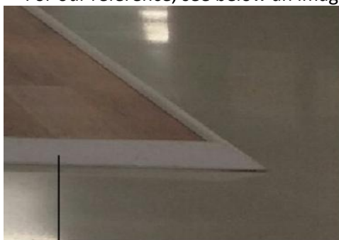
Raised floor (4cm) with sloping edges, finished with wooden laminate.
